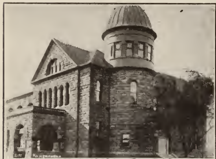
THE KAMEHAMEHA SCHOOL-BUILDING
